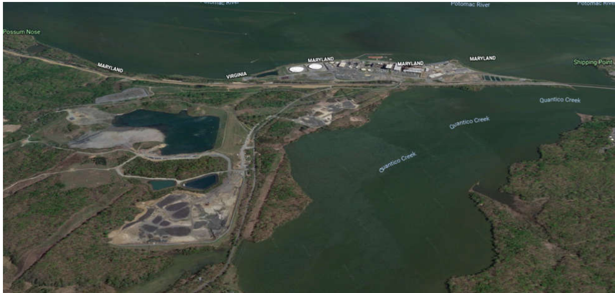
Figure 9 Possum Point Power Station (Image Google Earth © Google; Data SIO, NOAA, US Navy, NGA, GEBCO Google Landstat/ Copernicus)
