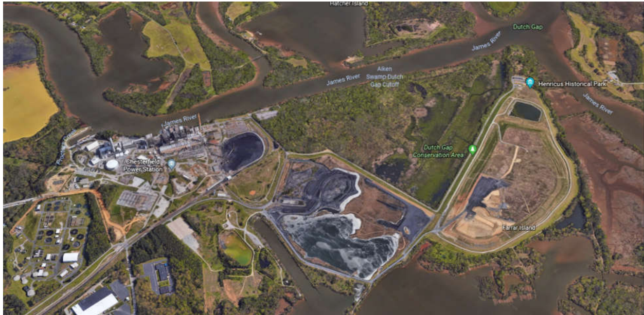
Figure 8 Chesterfield Power Station (Image Google Earth © Google; Data © Google)
