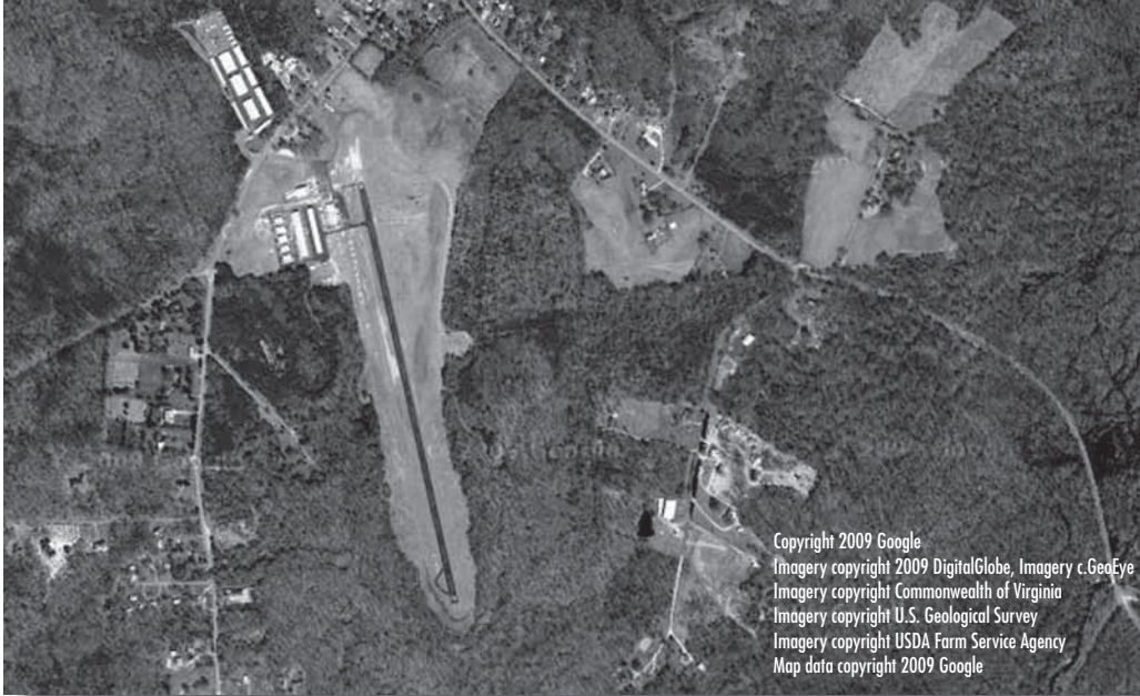
Aerial view of Maryland Airport near Mattawoman Creek
